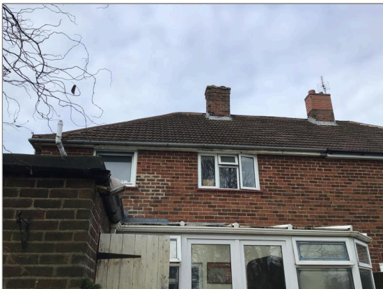
Photo - 2 Rear elevation
